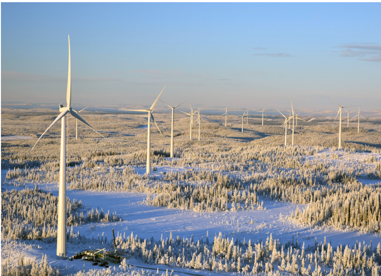
Figure 29. Frozen gas valve and a high-pressure pipe (© Nenets - Shutterstock) - top, and wind turbines operating in cold weather (© Feher Istvan - Shutterstock) - bottom.
