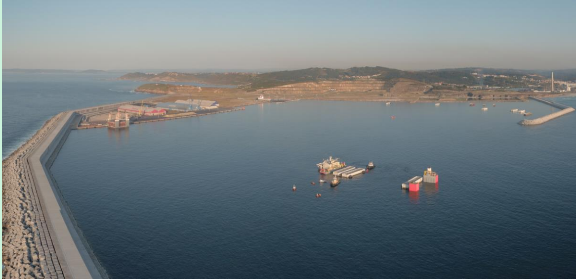
Figure 11. Shipment of concrete caissons leaving from the port of A Coruña
