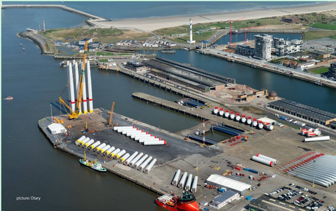
Figure 14. Tower Assembly in Renewable Energy Base of Oostende (REBO), Belgium (Courtesy of REBO)
